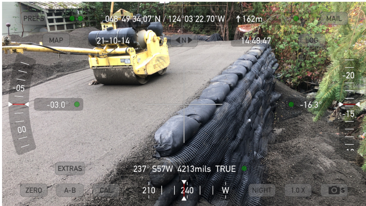
PHOTO #21.2 FINAL LIFT INSTALLED FOR REMAINDER OF SITE
