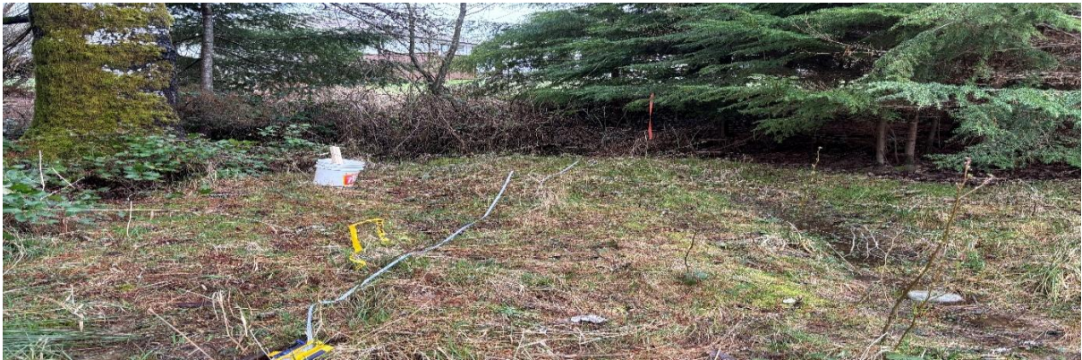
Little unnamed ditch starts here (orange flag) at the back of lot 20 (civic #216 Johel Road) & lot 21 (civic #224 Johel Road). rooftop storm water flows from these houses to this little ditch.
