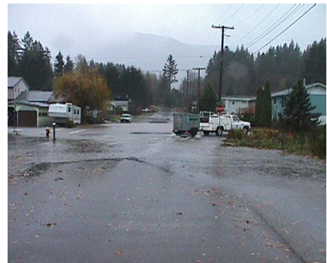
Frequent flooding at corner of Cowichan and Pine Street due to inadequate drainage
