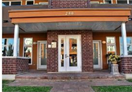
Figure 8 from the OCP: weather protected entrance
