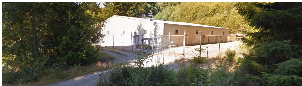
Figure 16 Water Treatment Facility on Indian Road
