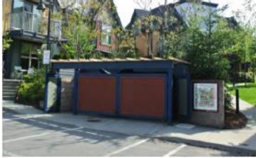
Figure 26 Example of screened waste enclosure
