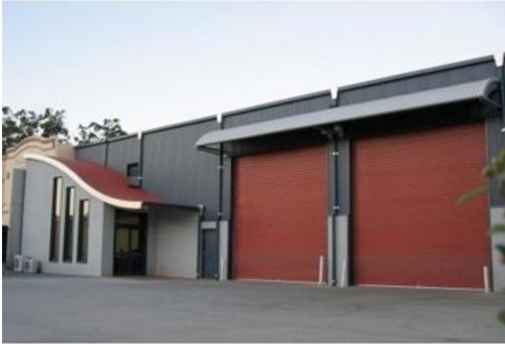
Figure 28 Articulated and varied roof lines
