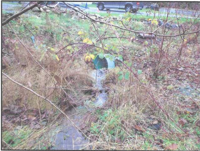
Looking downstream at the inlet of the culvert that conveys water off the subject property and into the stormwater system under Point Ideal Drive.
