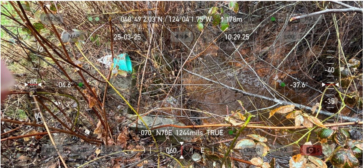
Figure 8. Green Culvert is below the subject property.
