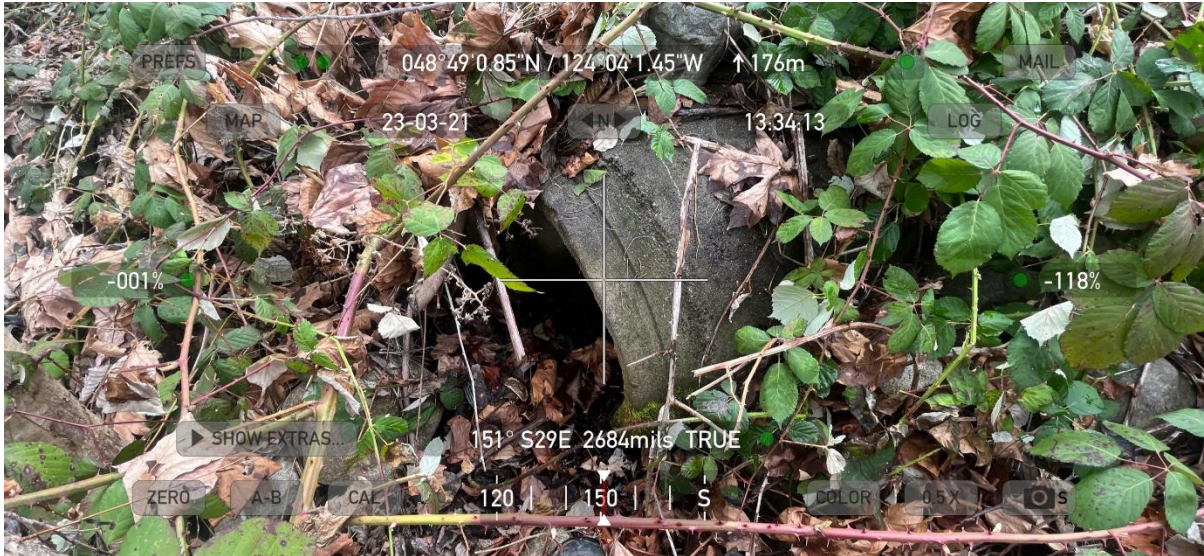
Figure 5. Upper 24" concrete culvert.
