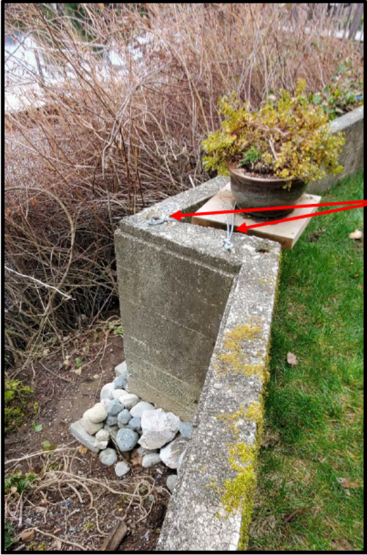
Images (Let & right) showing use of small chain and anchor bolts to keep retain wall together. Bank eroded at corner of wall.
