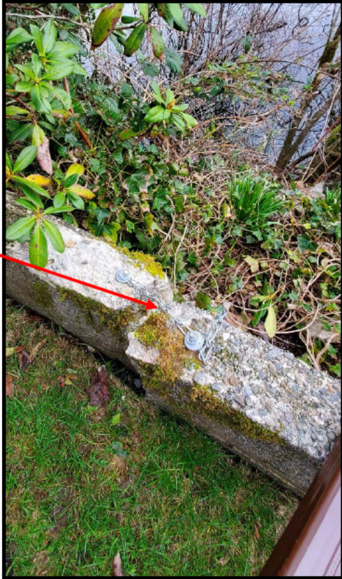
Images (Let & right) showing use of small chain and anchor bolts to keep retain wall together. Bank eroded at corner of wall.
