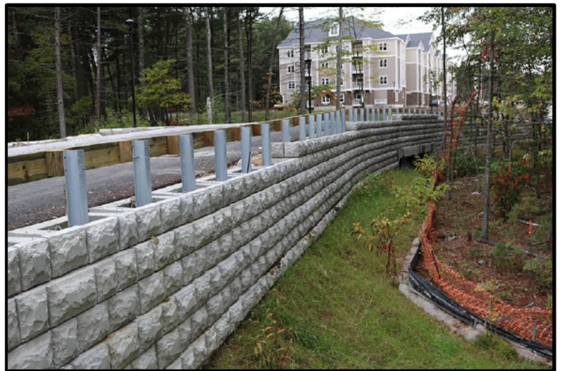
Example of stacked Verti-Block retaining use.
