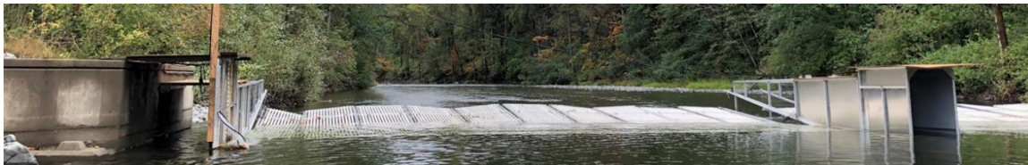
Figure 3: Two-passage counting fence configuration with wide passageways located mid-river and at the bulkhead, first piloted in 2019.
