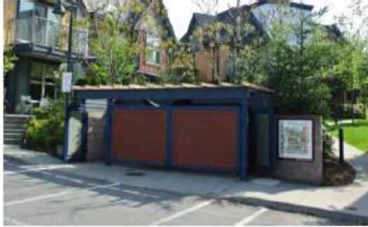
Figure 26 Example of screened waste enclosure
