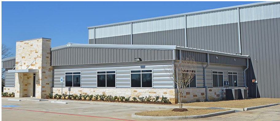
Figure 27 Use Concrete and Steel
