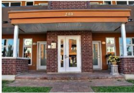
Figure 25 Weather protected entrance
