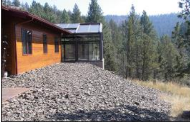
Figure 20 Fire break with no vegetation next to a house
