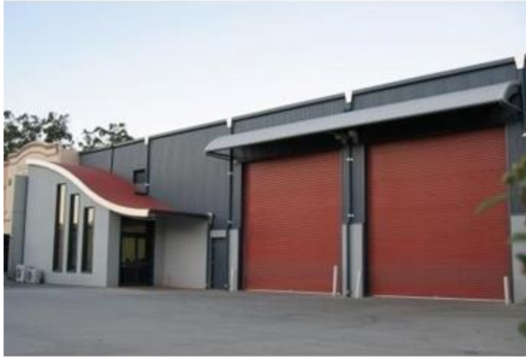
Figure 28 Articulated and varied roof lines
