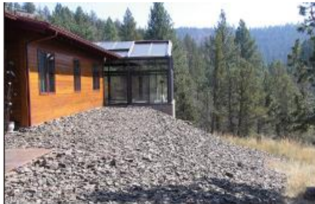
Figure 22 Fire Break with no vegetation next to a house
